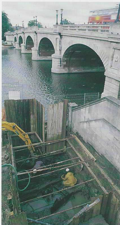
Kingston Bridge from the east, showing the proximity of the medieval revetment to the present river. The foreshore and banks of the Thames are together one of the richest archaeological resources in the London area
