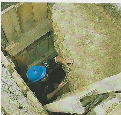
A small view of an enormous building: the foundations of the Roman basilica, one of the largest Roman buildings in Europe, were recorded beneath a former bank hall as it was being refurbished as a pub at 50 Cornhill in the heart of the City
