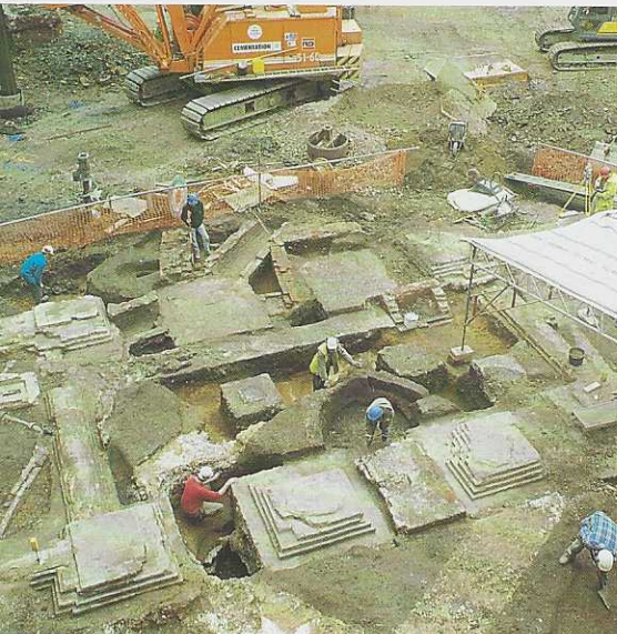
Lloyd's Register: masonry foundations of a 3rd-century Roman building are revealed in the foreground, punctuated at the same level by square brick foundations of Victorian buildings. This is often the case on City sites
