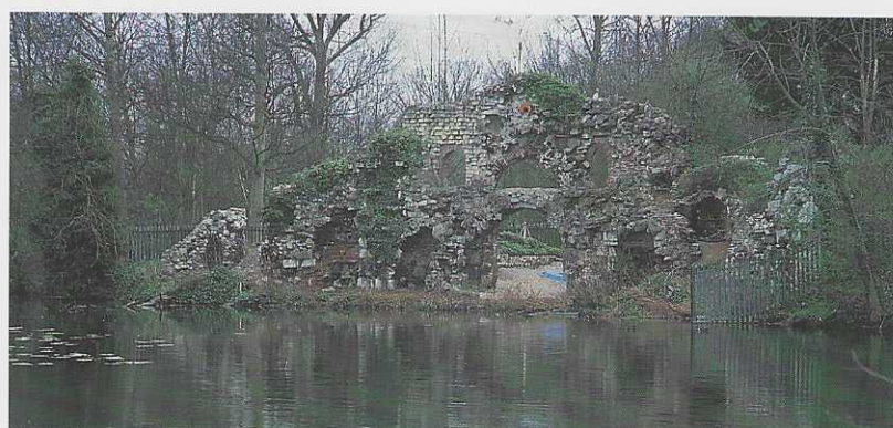
The north facade, partially restored, facing onto the Ornamental Water; the entrance arch to the boat dock in the centre
