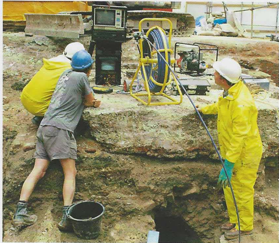
The first glimpse of the inside of the south end of the Roman culvert at Monument House, EC3, was provided by a CCTV survey carried out for us by the Corporation of London's Department of Technical Services.
