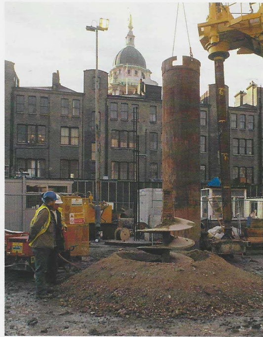
Monitoring the augering of new piles through the infilled medieval city ditch at the New Merrill Lynch Regional Headquarters, Newgate Street. The upcast from the piles contained numerous medieval artefacts including a decorated floor tile and a leather knife scabbard.
