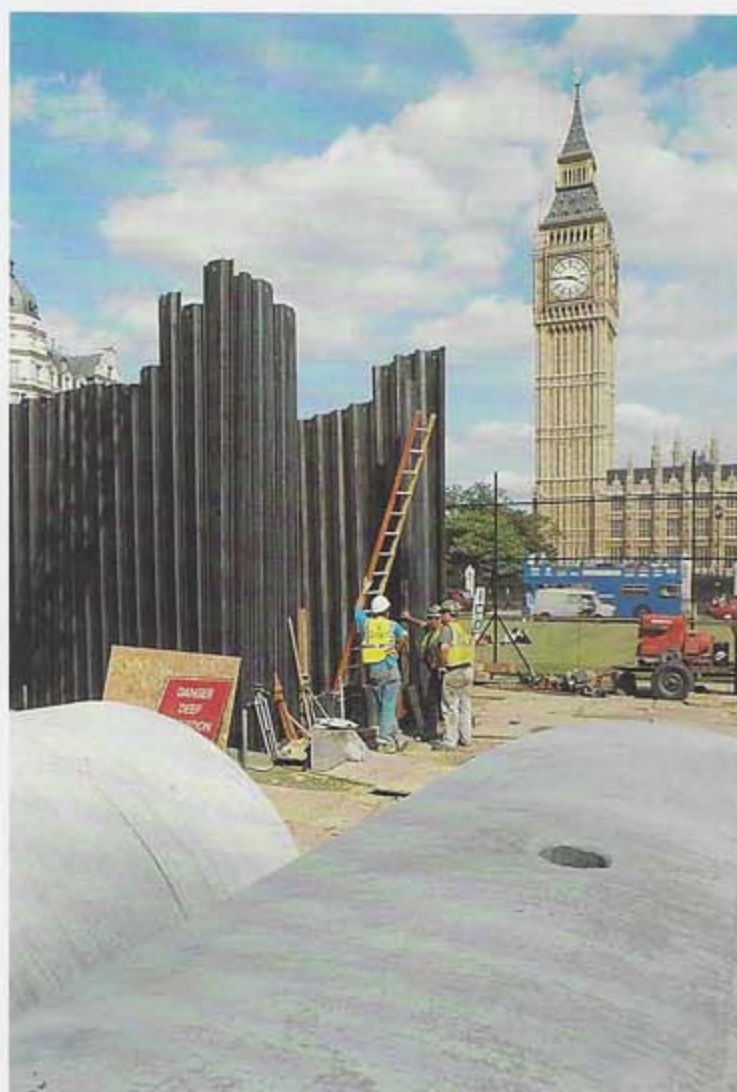
Above. General view of Parliament Buildings from the Jubilee Line excavations in Parliament square.
