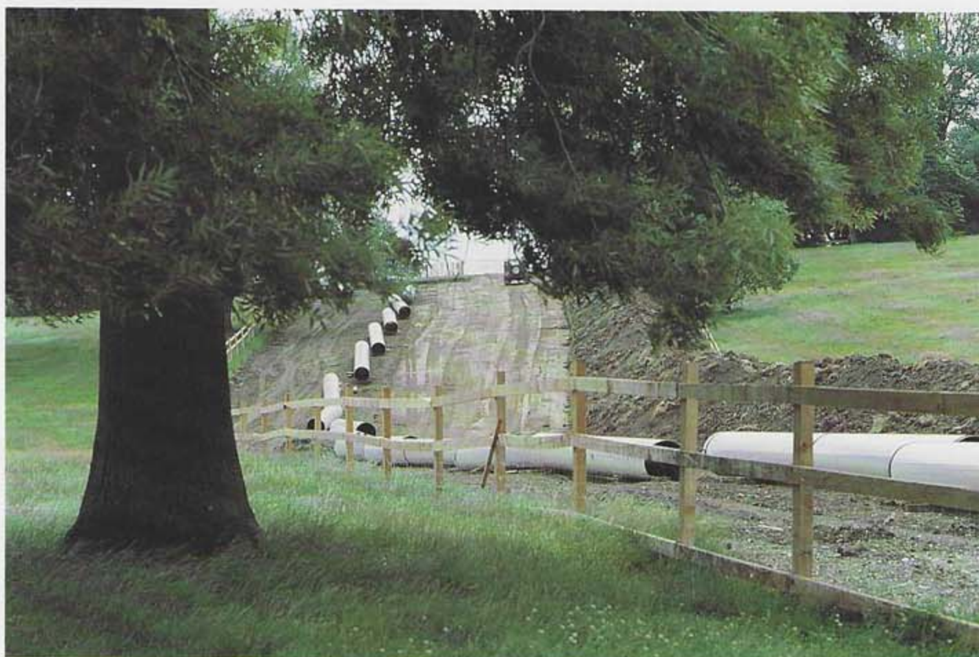
The British Gas pipeline crossing Hamstead Heath. MoLAS is involved with many major infrastructure projects such as the Jubilee Line extension and major road works and pipelines.
