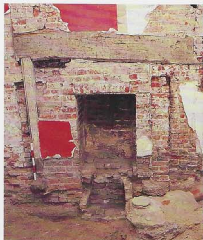
Sutton House. The kitchen in the east wing, showing the original 16th-century fireplace partially blocked by 18th-century brickwork.
