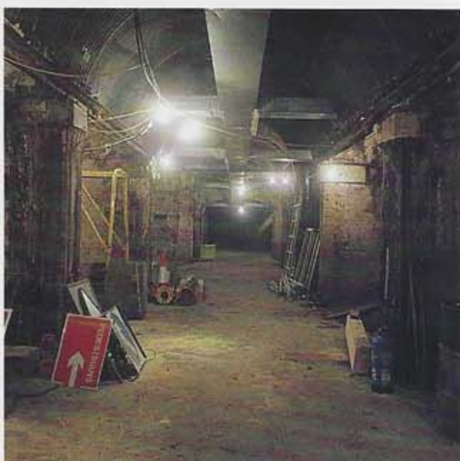
A general view of the excavation area of Mayor Swarder's Arches under the approach to London Bridge British Rail station.
