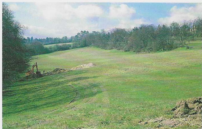
A23 Coulsdon Road: a view looking south across Summer Field, showing the trench cut to evaluate the ancient landscape, ahead of a relief road
