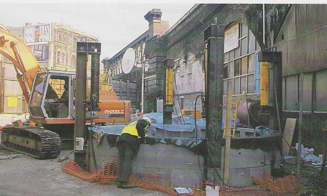
O'Meara Street, SE1: the top of the grout shaft, in which 3rd-century Roman buildings and the Roman foreshore were discovered
