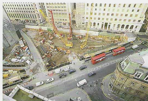
The site of Number 1, Poultry, from above, with Cheapside to the top of the picture. The insertion of perimeter piling is being monitored by MoLAS archaeologists. Excavation of Saxon and medieval streets, such as Bucklersbury (on the left), will follow
