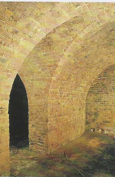
One of the vaults beneath Regent Street, recorded on the 172-182 Regent Street site; probably a part of Nash's building
