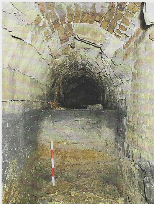
Internal view, looking north-west along the Great Drain of Westminster Abbey, found under the Jewel Tower garden
