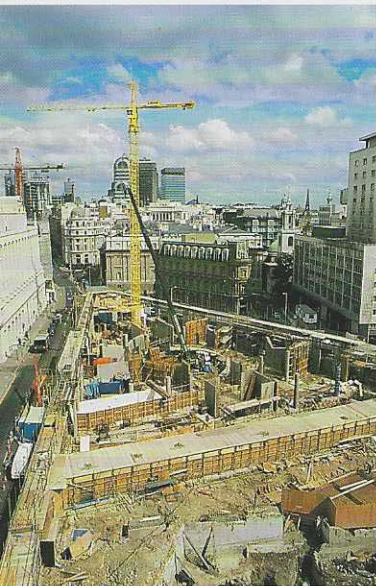
Aerial view of the site of Number 1 Poultry looking east. The cross section below shows how the excavations of the medieval and Roman remains proceeded whilst the building was constructed above the present street level
