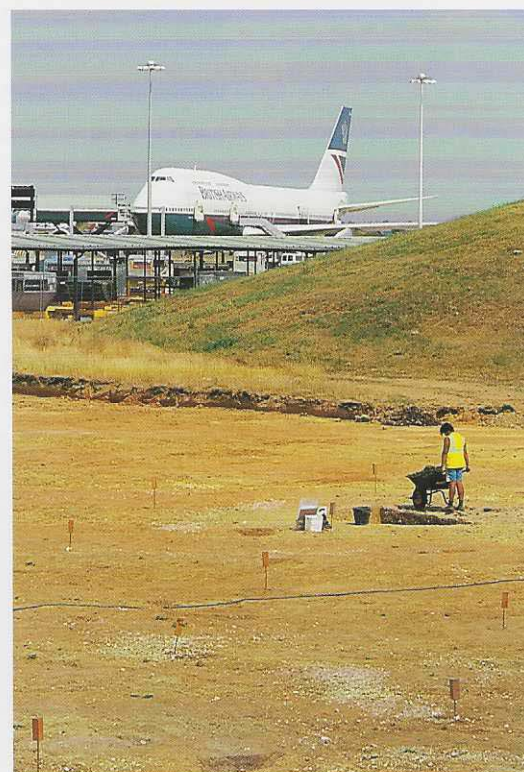
Extensive open area excavations underway to the west of the Terminal 4 jet stands at Heathrow Airport
