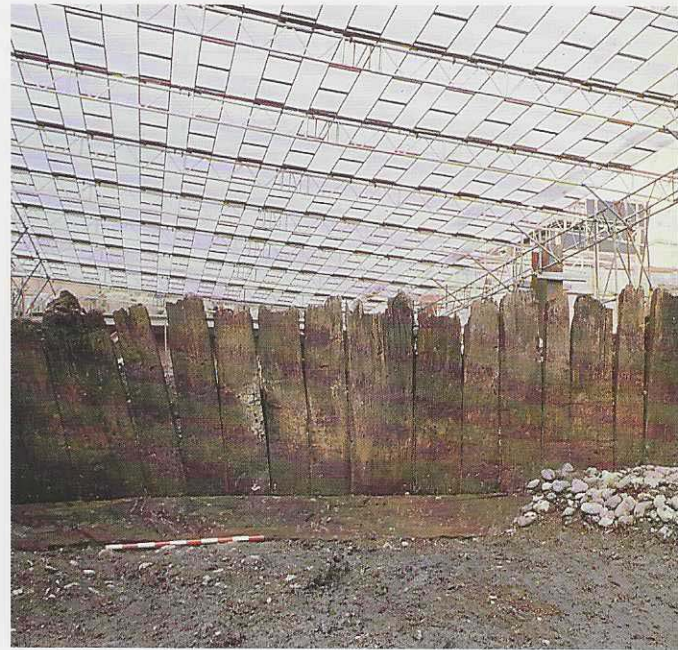
This stave revetment was constructed in 1121. The cobbles to the right were part of an earlier barge bed which remained in use, and have been partially removed to expose the revetment baseplate
