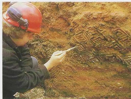
Roller-stamped chevron decoration applied on clay render, over mud brick, for keying plasterwork within the early Roman quayside warehouses
