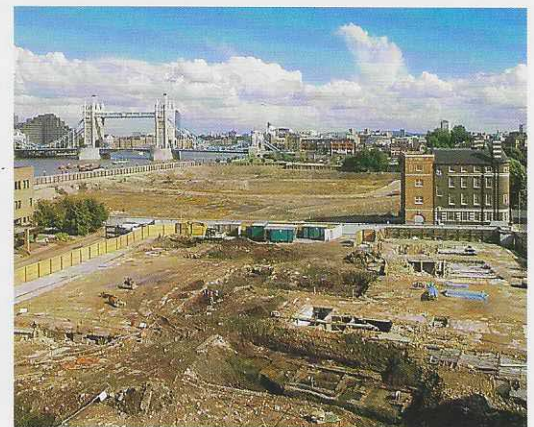
Overview of the site at Battle Bridge lane from the west with Tower Bridge in the background
