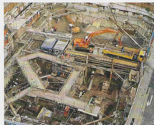
Regis House, autumn 1995, during the excavation of the early Roman harbour complex (foreground). Construction works are underway on the areas where excavation has already been completed
