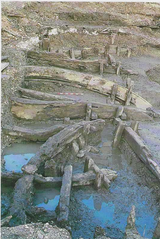
Looking north-east at the 17th-century ships' timbers at Bellamy's Wharf reused as land ties for a dock inlet and river wall. The curved white-lead painted timber is a virtually complete stem from a large ship very similar to that of the Vasa , the famous 17th-century warship now on display in Stockholm
