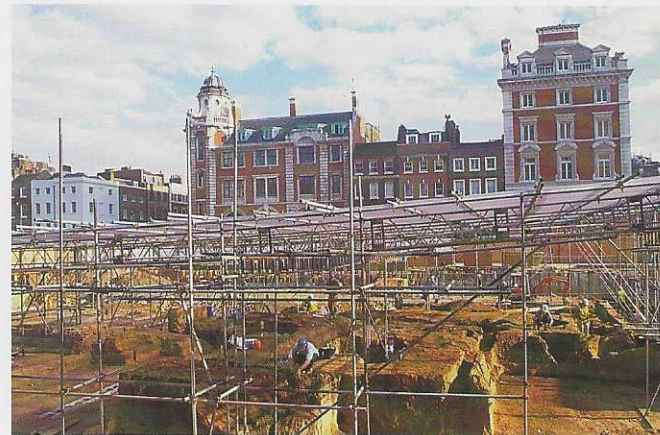
Over a four-month period an impressive sequence of buildings, pits and roads was recorded in advance of construction for the new Opera House scenery store
