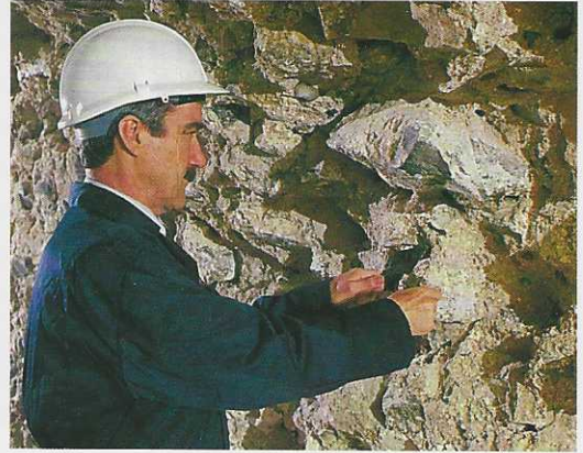
Inspecting the inside of Wren's foundations, exposed in the new tunnel. A small section of the foundations will be visible behind a panel in the tunnel
