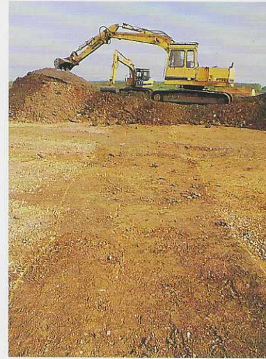
A ditch of the Stanwell Cursus prior to excavation at Perry Oaks Sludge Works
