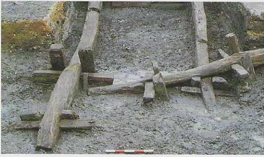
A detail of the landward tie-back braces for the revetments at Victoria Wharf
