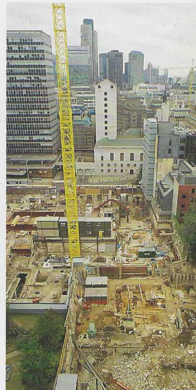
The excavations at Shelley House, looking east towards Wood Street
