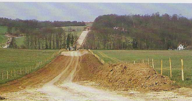
Part of the works on the North Downs Crossing section of the Channel Tunnel Rail Link, near Chatham (Kent)
