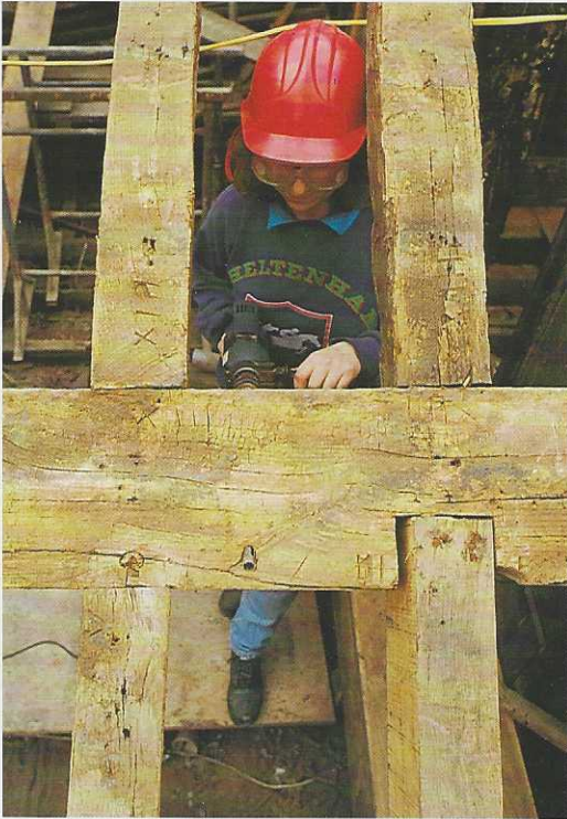
The recording work on the Gate, working from the accurate basis of plans and sections originally drawn by the architects for their own conservation work, studied the sequence of decoration of the panelling by sampling the layers of paint, and took samples for dendrochronology from the roof structure
