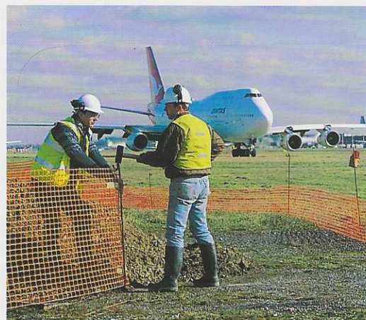
Preparing a site adjacent to the taxiways at the west end of Heathrow Airport
