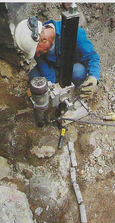
Diamond drilling in progress at Benbow House
