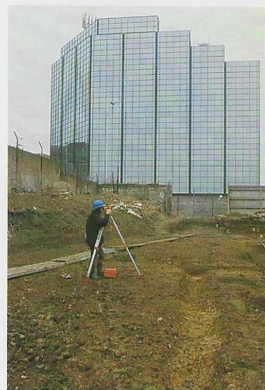
The modern surroundings of the excavation at Uxbridge High Street
