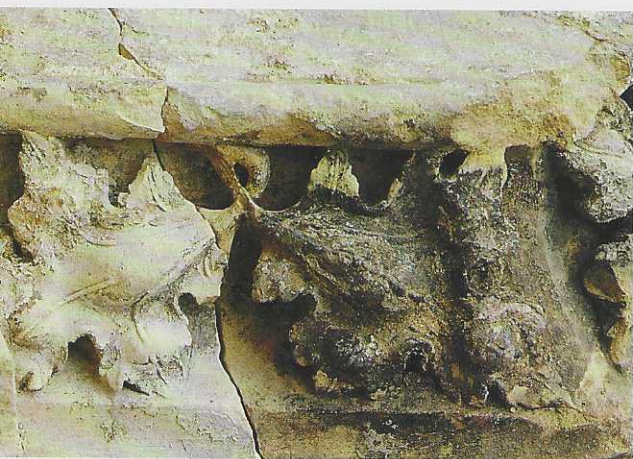
In the foundations of George Dance's porch facade of the late 18th century were a number of well-preserved medieval carved stones. These derived from the early 15th-century Croxton porch facade which was demolished to make way for the new work. The group includes part of the decorated blind panelling of the frontage, arch mouldings, and a (?) statue plinth, a detail of which is shown here
