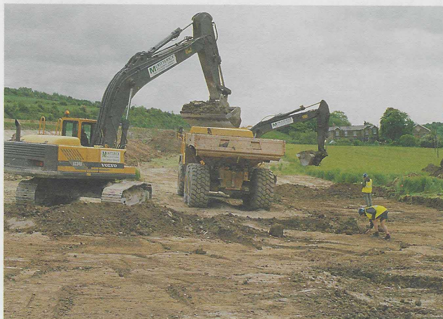
Topsoil being stripped in advance of archaeological work along the route of the A2/M2 widening
