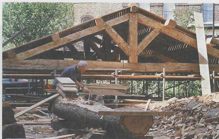
Full-scale replica of one of the late 1st-century buildings from Poultry, under construction for the display
