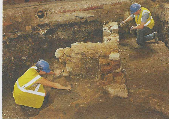
The masonry walls of a late 2nd-century building were found during the pre-demolition phase of work at Lion Plaza, during the excavation of foundations for temporary works designed to support the facades of Victorian banking halls being retained in the new development
