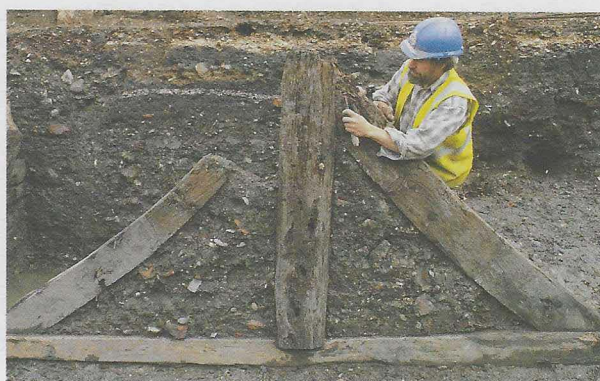
Ryszard Bartkowiak cleaning part of an 18th-century trestle foundation which included ship timbers, found at 165 Rotherhithe Street
