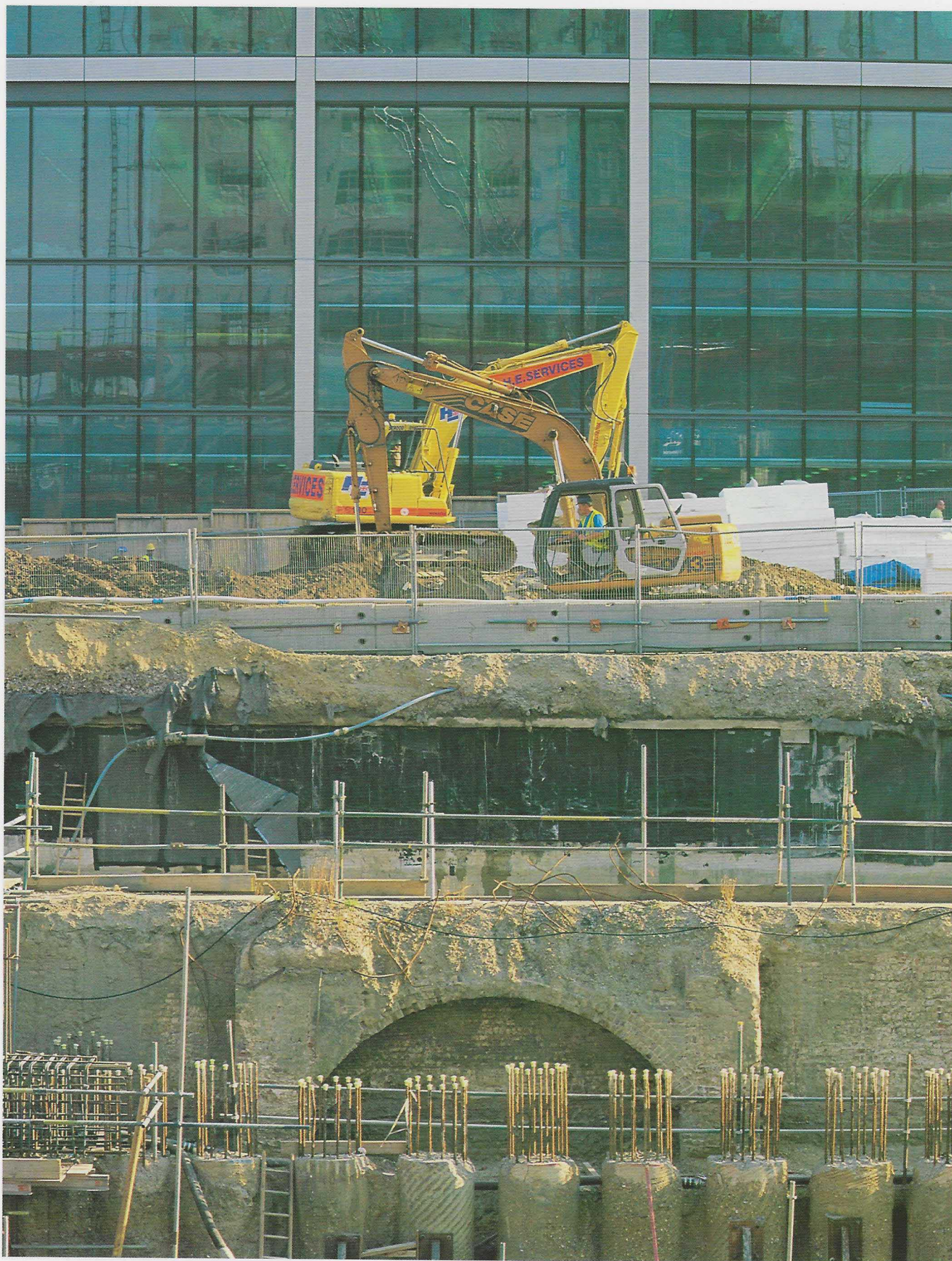
MoLAS archaeologists were surrounded by construction work at West India Docks, Canary Wharf
