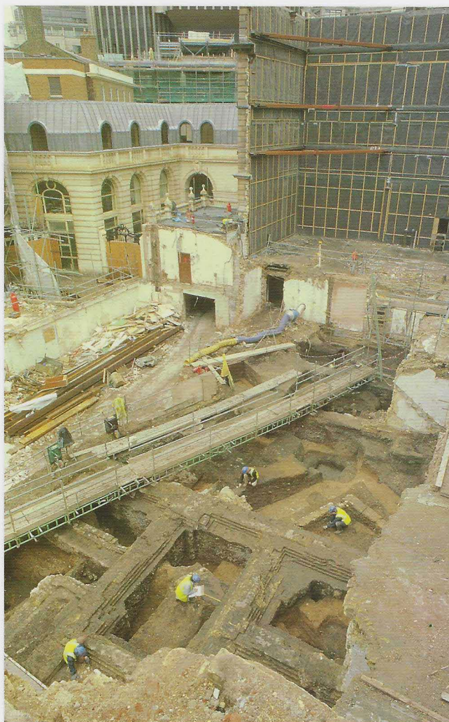
View of the second phase of excavations at Lion Plaza, which took place behind the retained facades of Victorian buildings
