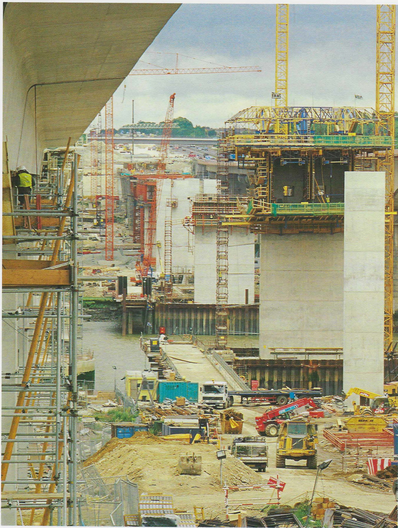
View across the Medway between the new Channel Tunnel Rail Link bridge and construction of the A2/M2 crossing, as construction work progresses
