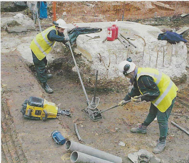
Levering the power auger out of the ground at Newgate Street
