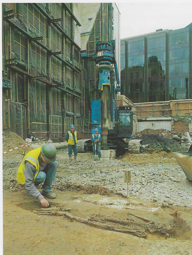
Excavating late Roman burials at Premier Place, Houndsditch, just outside the City wall
